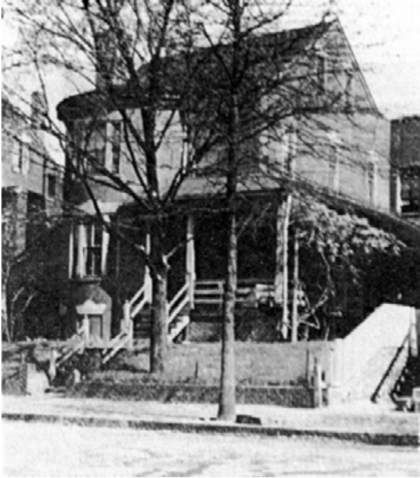
The Carrington House before restoration.
